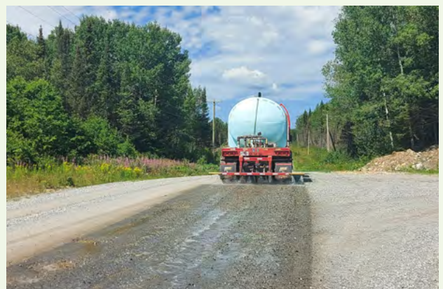
Application of dust suppressant
