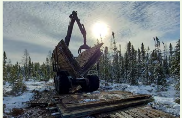
Wood mat installation to protect soils and vegetation
