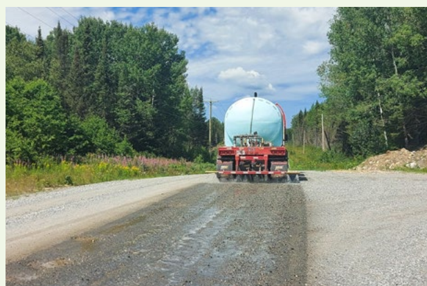
Application of dust suppressant
