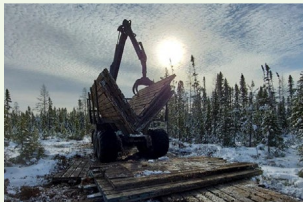
Wood mat installation to protect soils and vegetation
